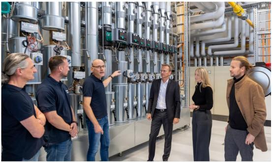
In a unique process Flender uses the waste heat from its hardening shop to heat the site in Bocholt. This saves almost 2.4 million kilowatt hours of natural gas and emits 400 tons less CO<sub>2</sub>.
